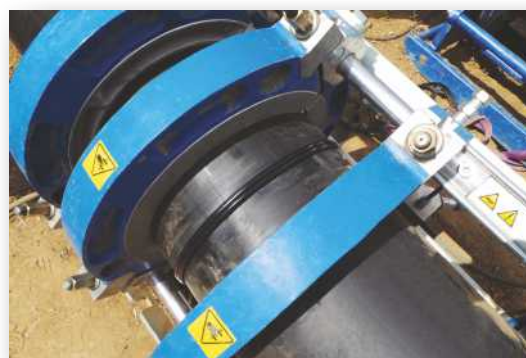
Unacceptable connection of pipes
